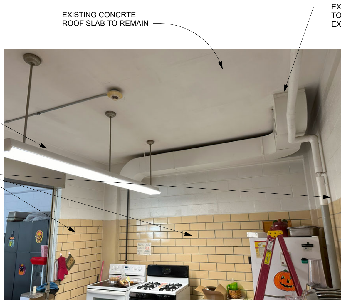
6 Existing Conditions Photo 3/8" = 1'-0"
