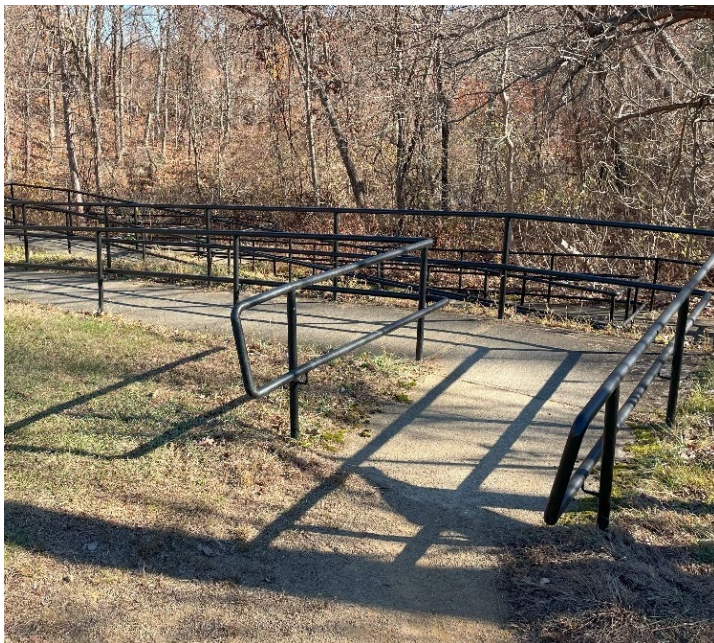
ADA Ramp to Heritage Trail Located at West Street Recreation Area
