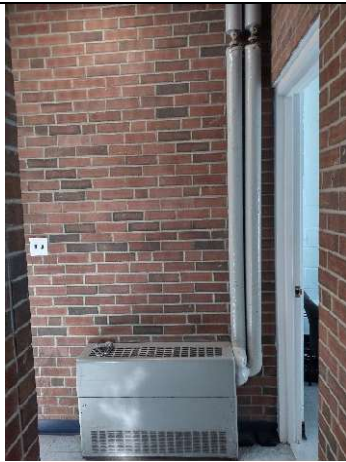
FCU front office hallway.
