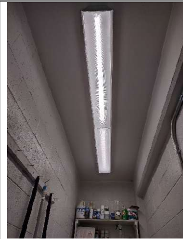
Typical traditional lighting. These tend to provide more glare since they do not “disperse” the light but rather simply shine down. The fixtures appear to still be incandescent and fluorescent type.
